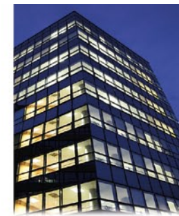
Before Daylight Cleaning
